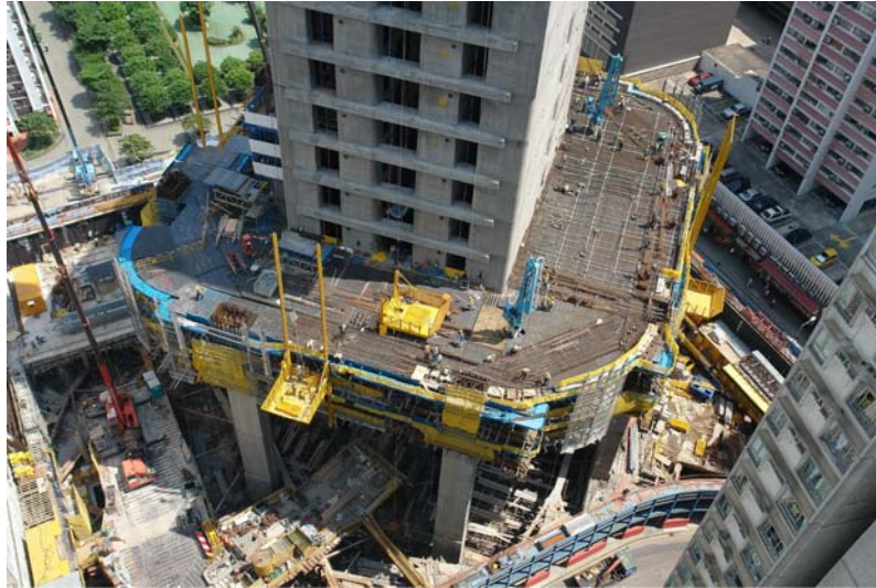
Figure 11. Virtual Simulation of the Build Methodology Optimizes the Actual Construction (Courtesy of Gehry Technologies)
