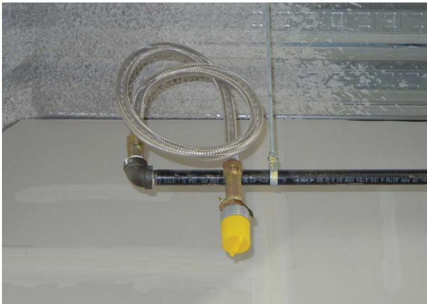
FIGURE 13.2 Flexible sprinkler head. © Howard Ashcraft.
