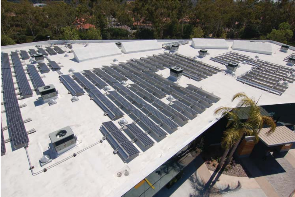
FIGURE 6.9 Rooftop equipment to reduce use and produce energy. © DPR Construction, by David Cox.
