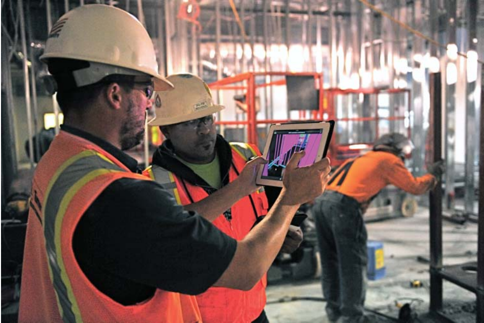
FIGURE 10.11 Field foreman looking at BIM for framing and in-wall utilities details. Licensed by The Regents of the University of California on behalf of its UCSF Medical Center; courtesy of DPR Construction; courtesy of Mirror Mirror Digital Media, Inc.
