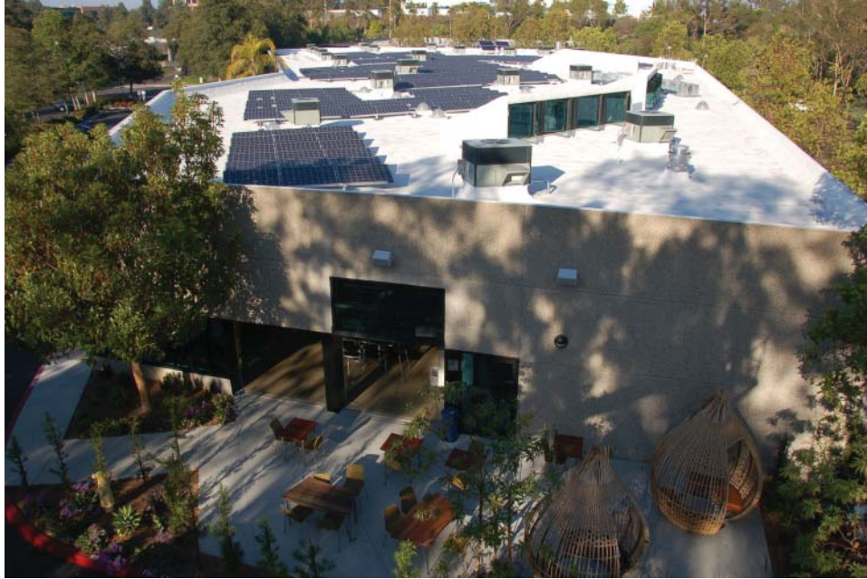
FIGURE 6.8 A greener, more permeable site and an energy-efficient rooftop membrane. © DPR Construction, by David Cox.
