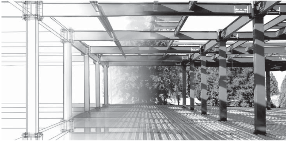
FIGURE 7.7 From BIM to reality using the ConXtech modular system. © Yong Chan Kim, ConXtech, Inc.
