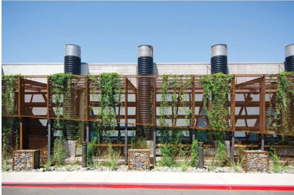
FIGURE 4.6 Shower towers (black columns), green screening, and operable windows. Gregg Mastorakos; courtesy DPR Construction and SmithGroupJJR.
