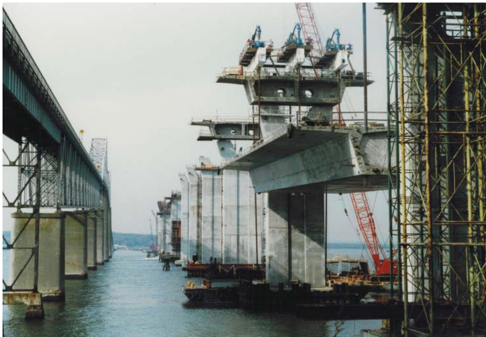
FIGURE 1.1 Prefabricated box girder deck being set in place. Courtesy of Michael Veegh.
