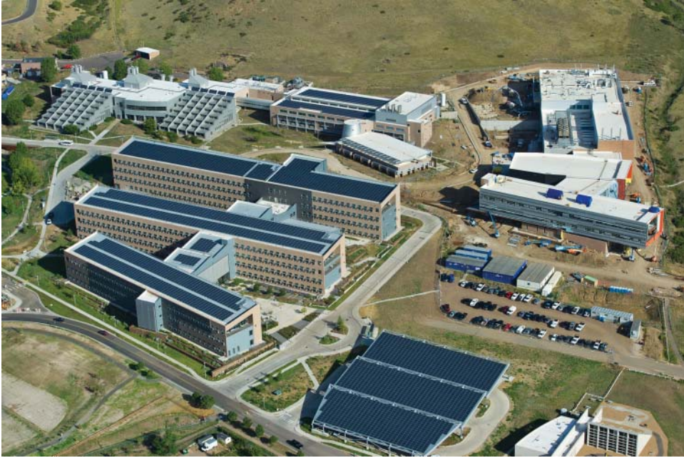
FIGURE 4.10 Aerial view of the RSF buildings. Photograph by Dennis Schroeder, National Renewable Energy Laboratory, NREL.gov.
