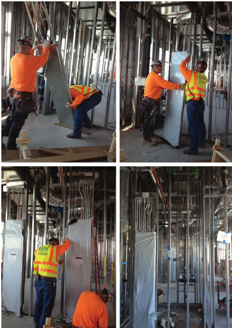
FIGURE 1.2 Headwall installation. Licensed by The Regents of the University of California on behalf of its UCSF Medical Center; courtesy of DPR Construction.
